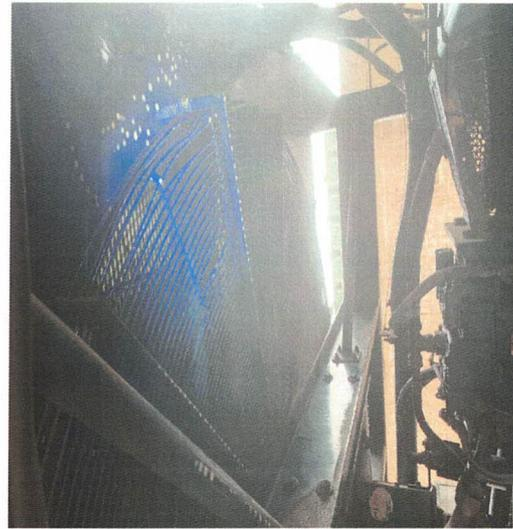
Fans and coolers end up getting covered in dust, then oil mist finds its way to adhere to the dust, which then sticks to fans and bearings, once the oil coated dust works into bearings the coolers have to be shut down and the bearings replaced.
