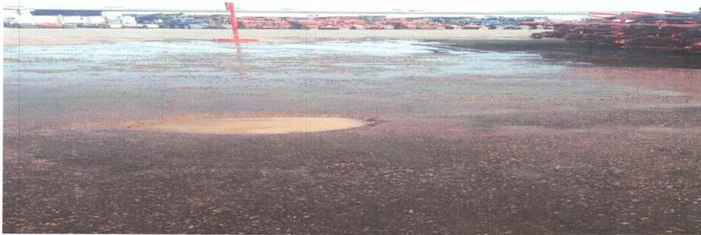
**This large concrete spill with gearbox oil, required 2 hours of applying OSE II, then 1 hour of rinse down, and the entire surface was free of gearbox oil, and since OSE II lifts oil/hydrocarbons out of the pores of the concrete the surface was no longer slippery as well. The effluent wash off will become CO2 and water, the environmental impact was reduced on contact with OSE II.**
